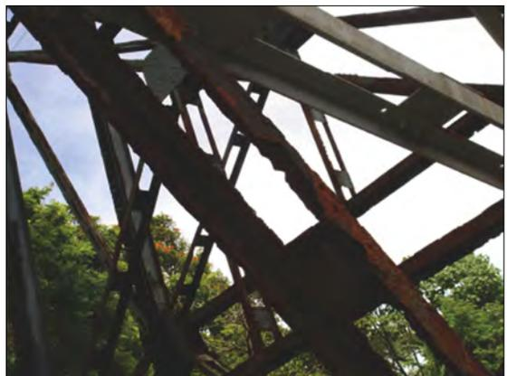
Weather permitting, spraying will begin at the end of February and continue in two phases. The process will consist of an initial inhibitor application, including time allowed for saturation to counter the buildup of corrosion scale, followed by a second application within hours of the first. The specification is to spray the bridge annually until the budget allows for the complete replacement of components, after which a conventional coating system will be put into place.
