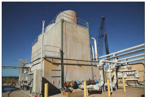
Testing of the walls showed corrosion rates between 16.72 and 67.91  $\mu\text{m}/\text{year}$ , which indicates a low to moderate level of corrosion.
