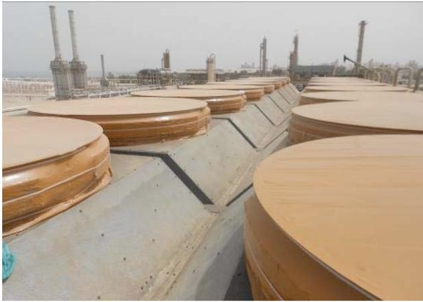
**The fin fans were coated with Cortec® coatings and covered with anti-corrosion MilCorr® film**
