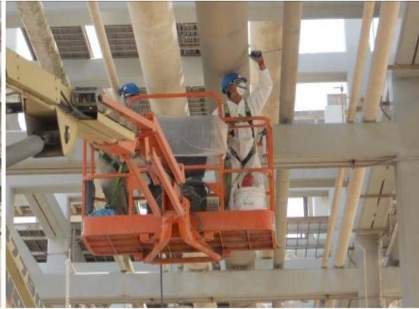
**Insulated pipes being injected with VpCI® inhibitor**
