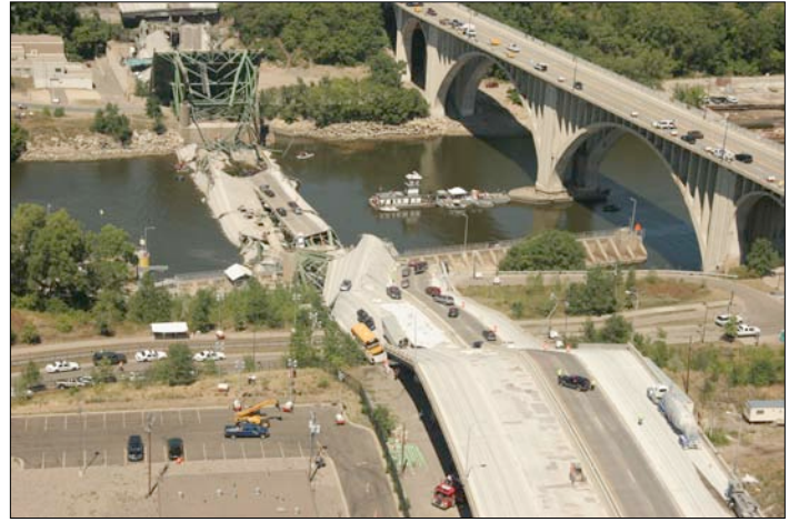
Minnesota 35W Bridge after collapse August 1, 2007.
